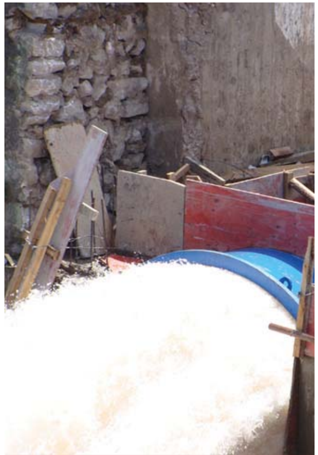
Optional hood discharges flow into confined areas
