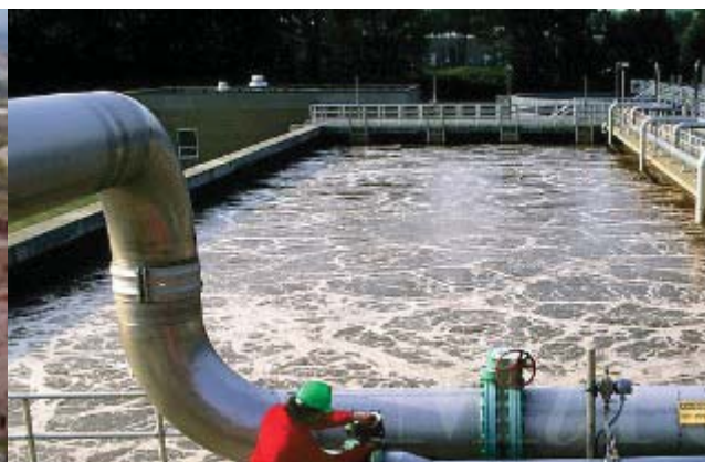
4 Sewage Treatment Plant
