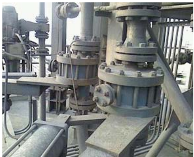
Installation on Job Site
