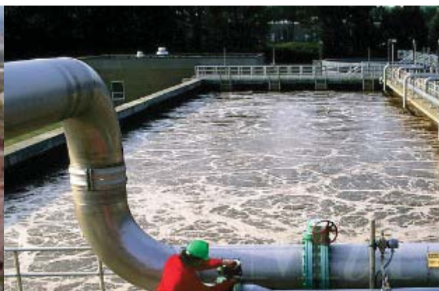
4 Sewage Treatment Plant
